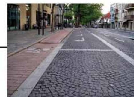
Treatment of road surface
