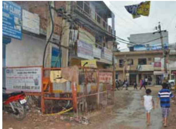
Transformer on the road
